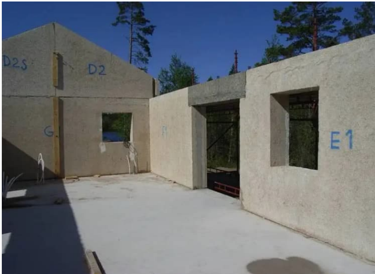
Figure 3.1—Home Under Construction Using WWC-LWE for Walls
