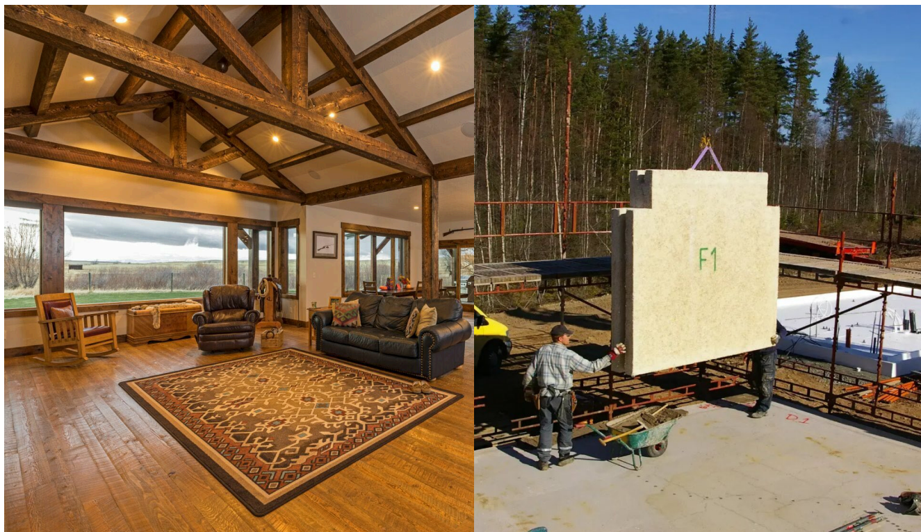
Figure 1.2—Example Large Dimension Timbers (left) and Wood Wool Cement Large Wall Elements (right)
